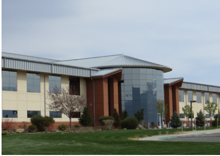
GE Bently Nevada anchors Douglas County's technology cluster.
